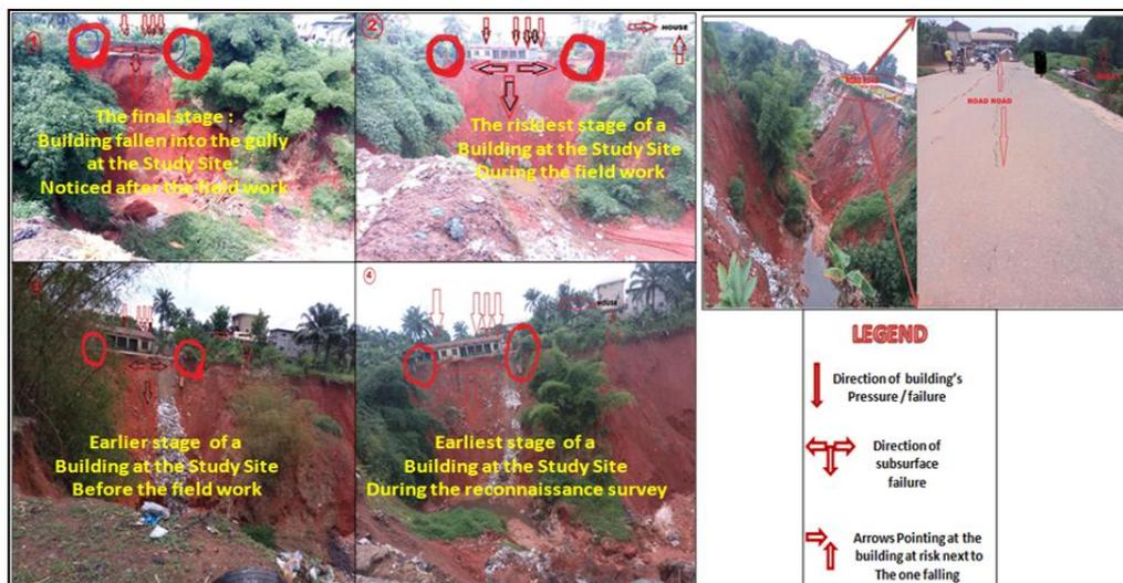
Figure 1b: Active and Progressive failure of a superstructures and a Major Road at the Uruagu-Nnewi Gully site
